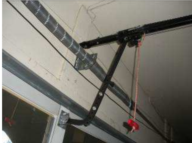
Photo 2: Door Lift Bracket Assembly
